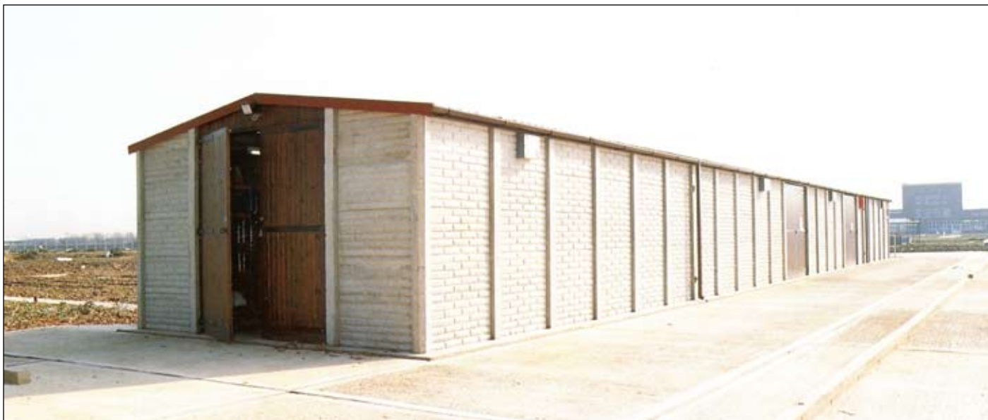
Amenities block for an allotment association in Slough, providing toilet facilities, storage and a shop.
